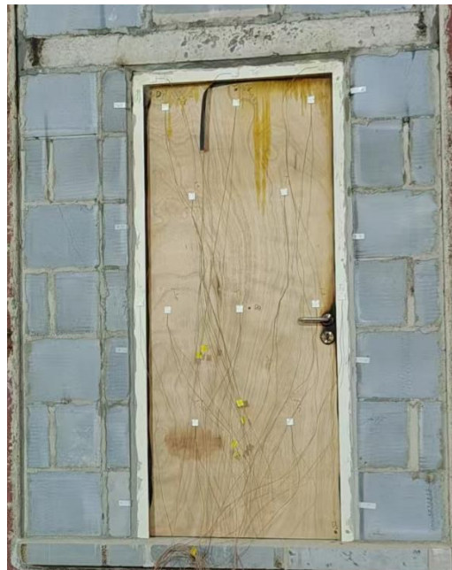
Fig. 6 Unexposed Side after 120 Minutes
