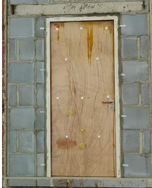
Fig. 3 Unexposed Side after 30 Minutes
