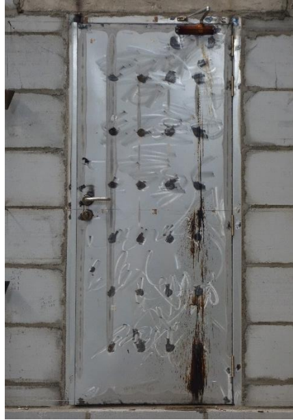
Fig. 3 Unexposed Side after 90 Minutes
