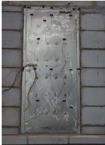
Fig. 2 Unexposed Side Prior to the Fire Test
